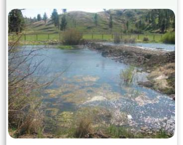
This type of artificial beaver dam, distinguished in the rulemaking as a "restoration check dam," is made from rocks and dirt and generally does not involve real beavers. Dams such as these may reconnect incised streams with their historic floodplains, but they also may block fish passage, and their impacts on stream flow and water temperature are not well known.
