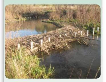
This type of artificial beaver dam, distinguished in the rulemaking as a "beaver dam analogue," is designed to mimic a real beaver dam, and help real beavers build their own dams in streams where channel incision has made dambuilding difficult. Dams such as these are generally thought to help watersheds by reconnecting streams to historic floodplains without overheating the water or blocking fish passage.
