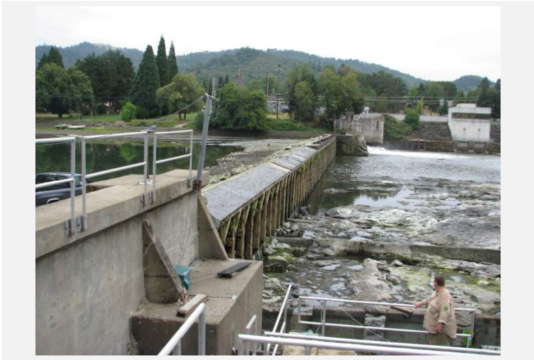
Figure A1-8: Downstream dam face during drawdown (09/01/2009)
