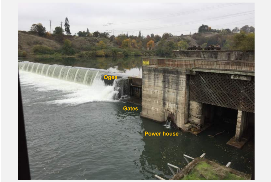
Figure A1-2: Powerhouse and gates, looking north (10/25/2017)
