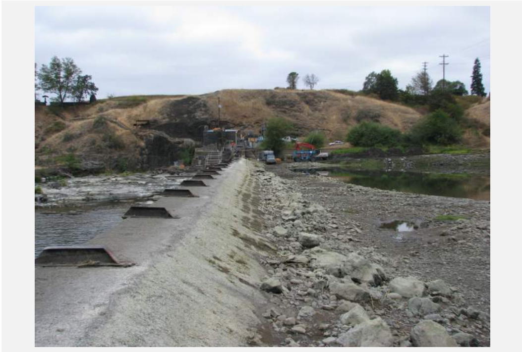
Figure A1-11: Upstream dam face during drawdown (09/01/2009)
