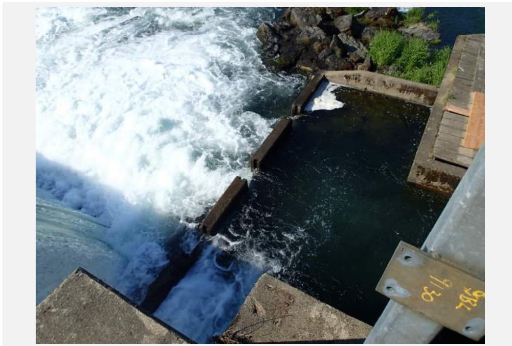
Figure A1-4: Fish ladder during normal operation (05/30/2019)
