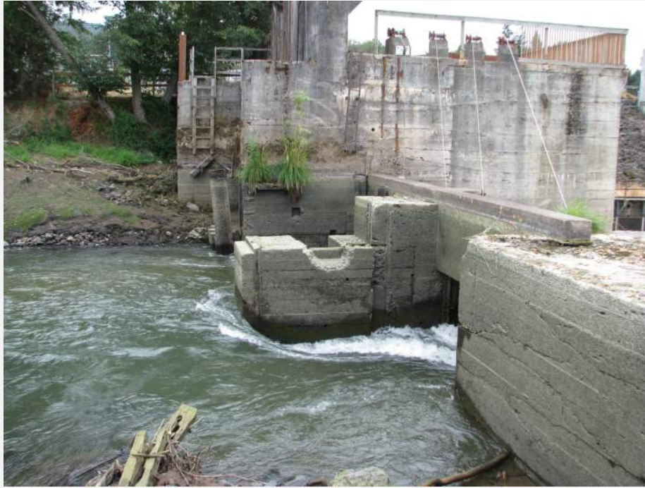
Figure A1-9: Upstream view of the gates during drawdown (09/01/2009)
