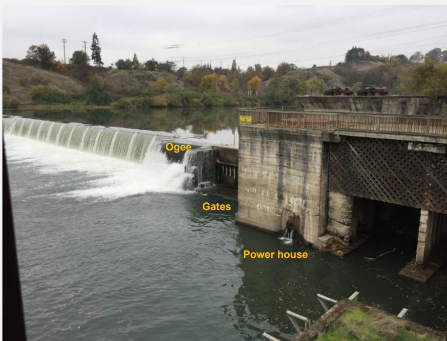
Figure A1-2: Powerhouse and gates, looking north (10/25/2017)
