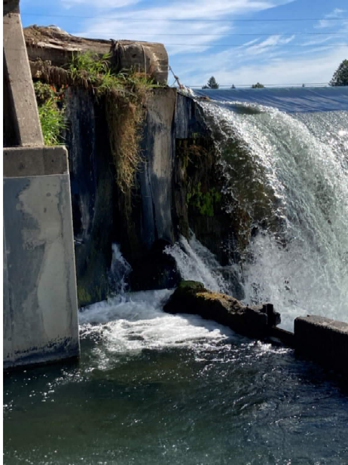
Photograph 5: View of the false attractant flowing through the dam (center of photo) near the fish ladder. (June 2021)
